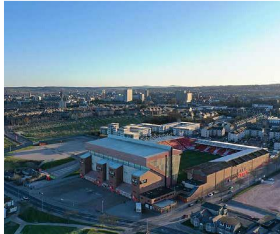
Aerial view of Pittodrie Stadium from the north east
