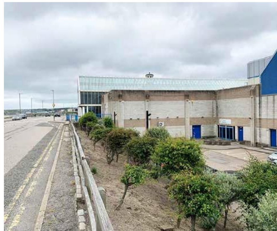
Existing Entrance and external facade
